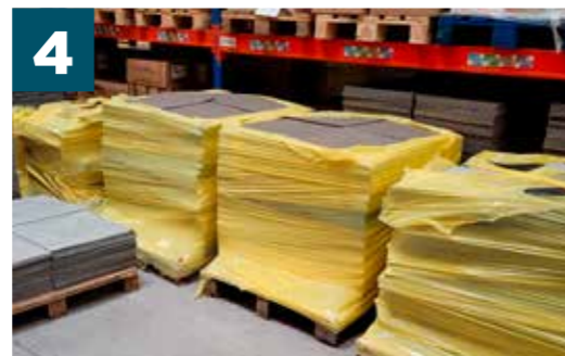
4 Disposal of non-reusable tiles for recycling*.
