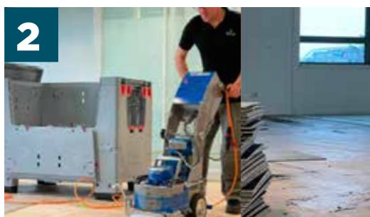
2 On-site cleaning, removal and sorting of slabs suitable for re-use
